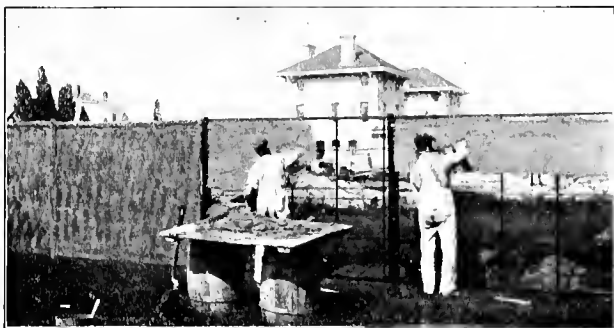
Fig. 139—Progressive Operations in the Making of a Cement Mortar Fence
